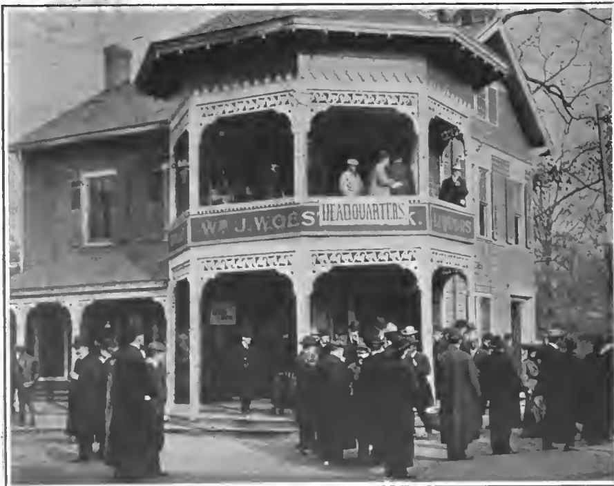
HEADQUARTERS AT FOOT OF HILL—OFFICIALS IN VERANDA BALCONY CAN SEE TAPE SHOWN ON PRECEDING PAGE.
